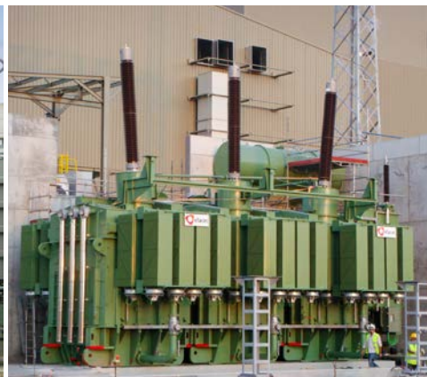
Three-phase GSU Transformer 508MVA, 416kV (Portugal)
