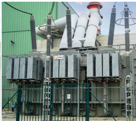
Three-phase GSU Transformer 528MVA, 410kV (Portugal)
